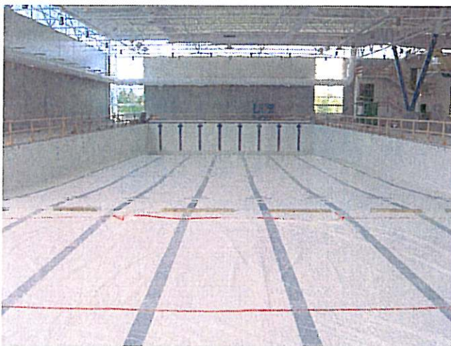
Figure 5: 50-metre pool with tiling in place
